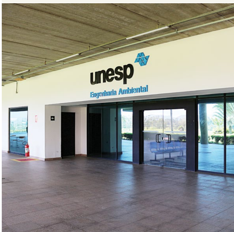
ICT_Unesp facade in PqTec
